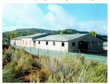
Exterior view of one of the four Camp Lockett buildings showing the badly deteriorated roof.
